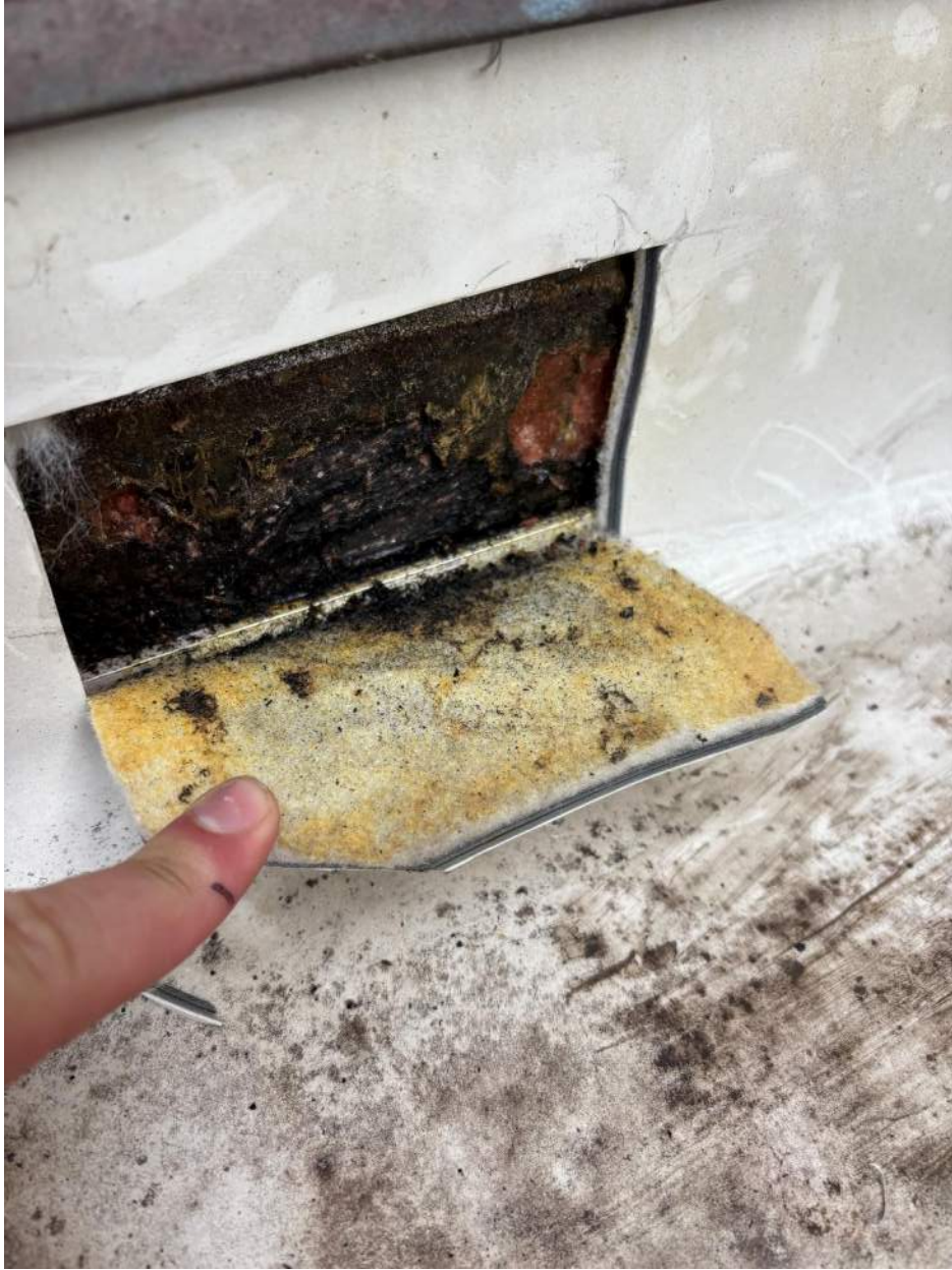
The last few photos show various curb cuts on the auditorium roof.
